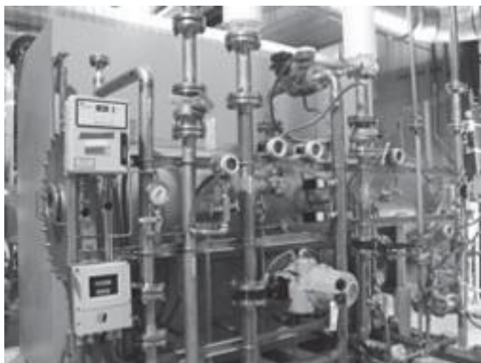
Figure 15.3 Ozonia Ozone Generator (S. Hanson photo file)
